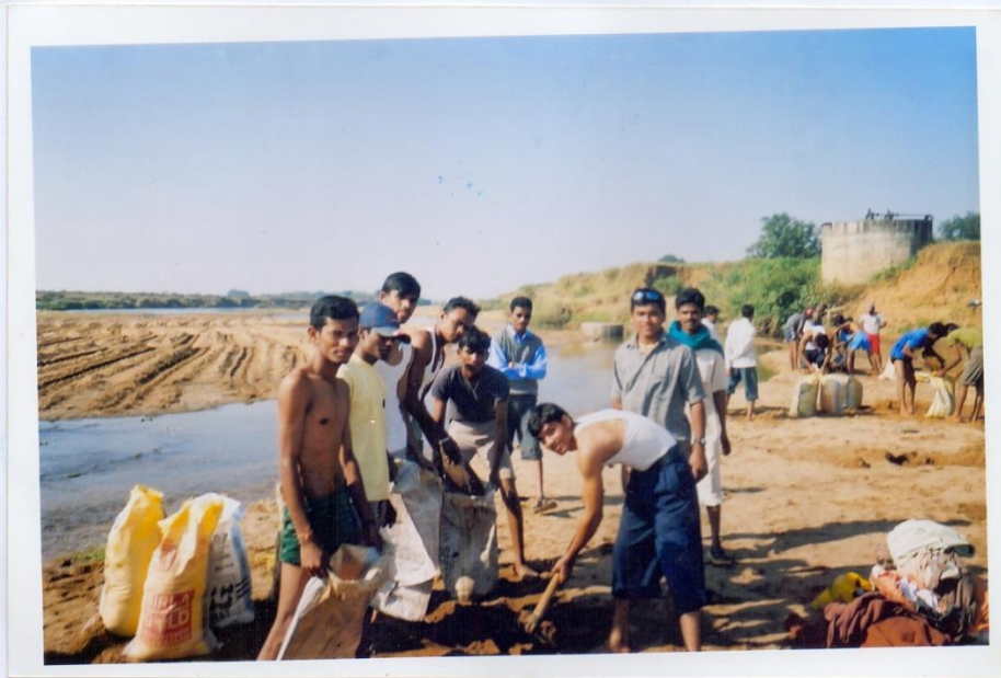
Sand Dam Built Developed on Kathani river by N.S.S. Unit.
